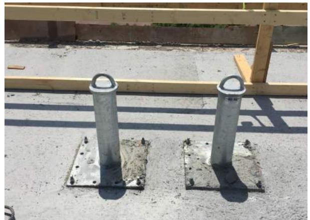
ES StrongTop Anchorage Connector Cast in Concrete
