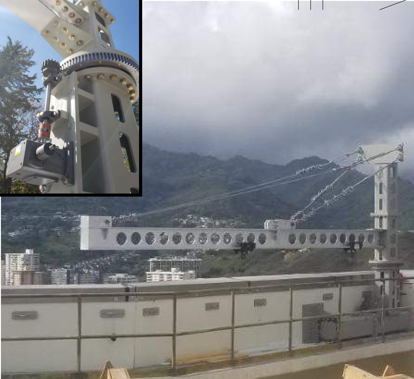
EXTRA LONG REACH DAVIT ARMS INCORPORATE POWERED DRIVES AND ARE USED FROM OVER 12'-6" REACH
