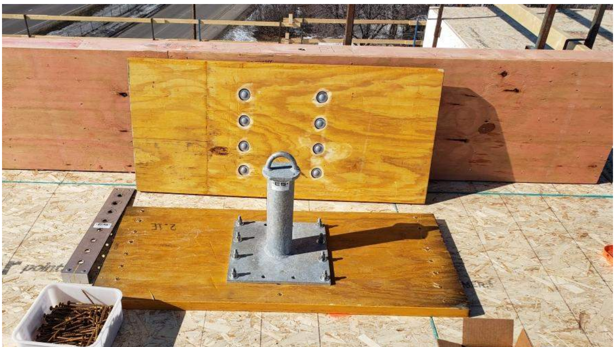
ES StrongTop Anchorage Connector on Wood Plinth
