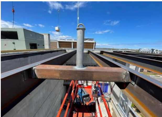
Engineered Supply StrongTop Anchor to Tube Spreader
