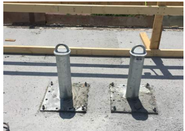
ES StrongTop Anchorage Connector Cast in Concrete
