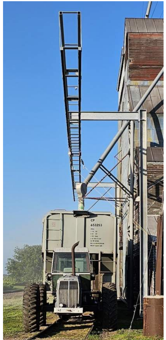
Dual Monorail Truss from Gallows Arms
