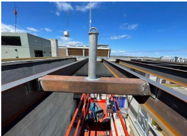
Engineered Supply StrongTop Anchor to Tube Spreader
