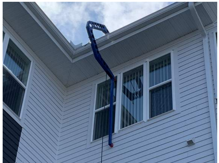
AROUND THE GUTTER PINNED OUTRIGGER LAUNCHED
