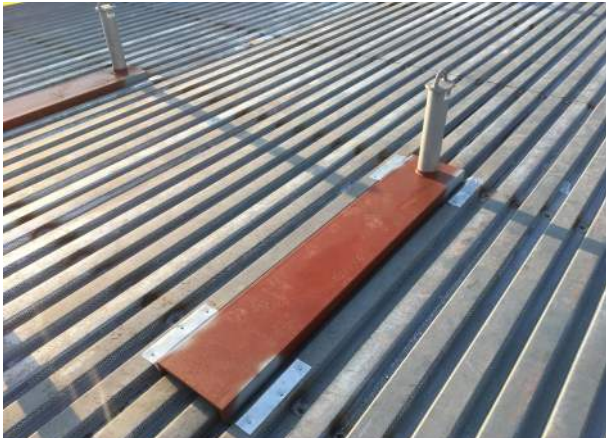
Engineered Supply StrongTop Anchor to Bar Joist
