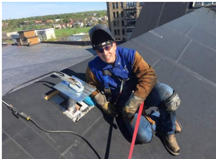
Engineered Supply StrongTop Anchor to Heavy Structural Steel Truss
