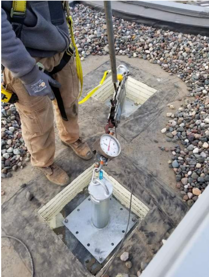
ES StrongTop Anchorage Connector Post Installed on Concrete
