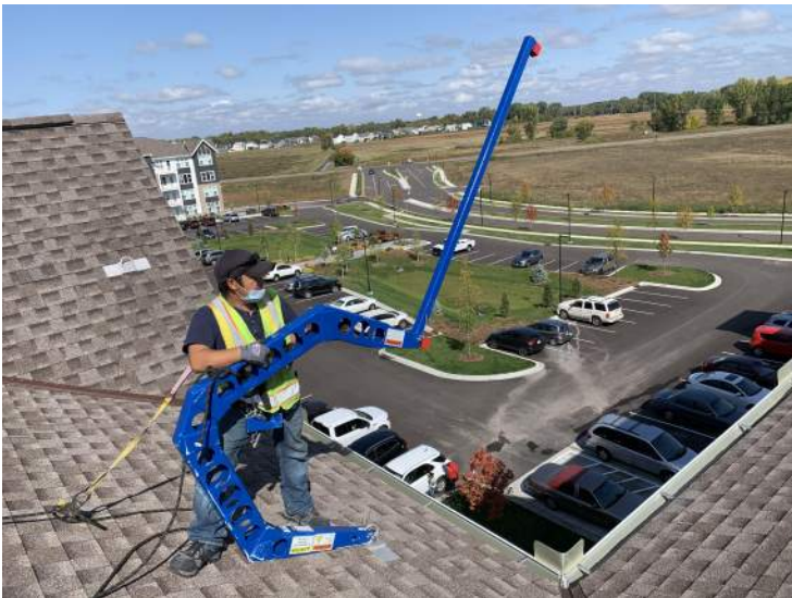
DOWN AND UNDER PINNED OUTRIGGER
