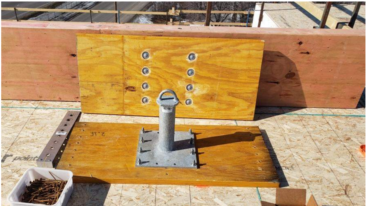
ES StrongTop Anchorage Connector on Wood Plinth
